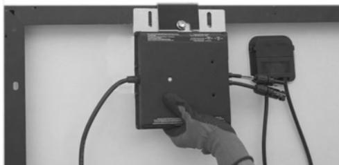
4. With a 13mm or 1/2 inch socket wrench, tighten the cap screw until you reach a torque of 18 Nm (13 ft-lbs).
