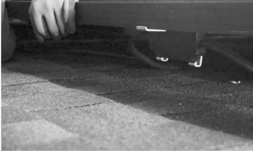
10. Secure the Engage Cable to the module frame with wire clips as needed.
