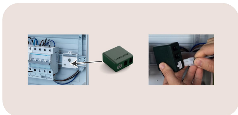
Image 4: View on a distribution panel with DIN mounting plate and Power Box
