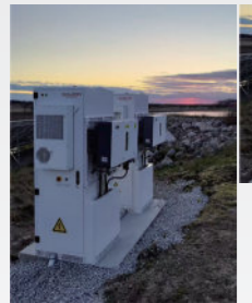
Sweden OASIS 60 & Solinteg 100kW/120kWh Outdoor Battery Cabinet System BESS for Small Solar Park
