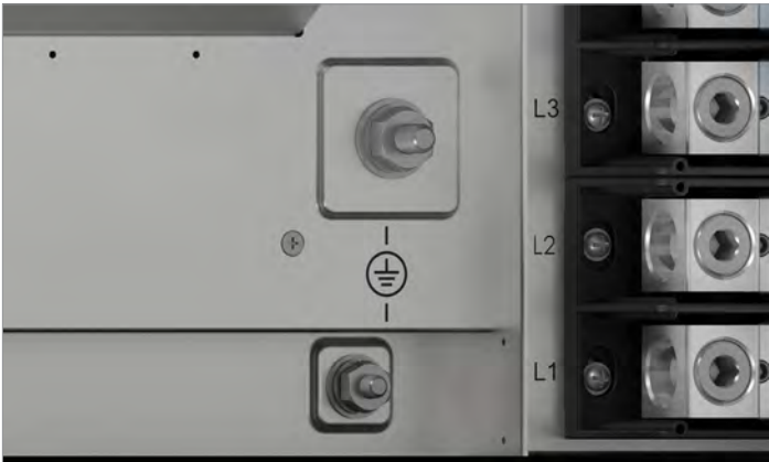
Abb. 6.19: PE-Anschlüsse
