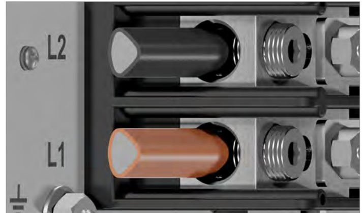
Abb. 8.13: Correct position of sector-shaped aluminum cables (2)
