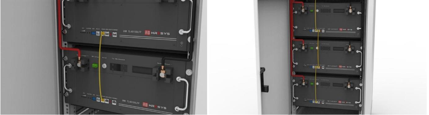
**Step 10: IMPORTANT !** Connect firmly each module's front panel to the 19" rack of the cabinet by earthing cable (as per picture below-left).
