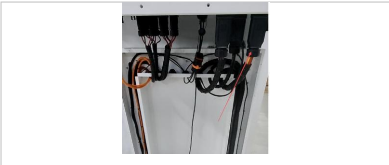
Figure 6-24 Connect the grid AC cable to PCS
